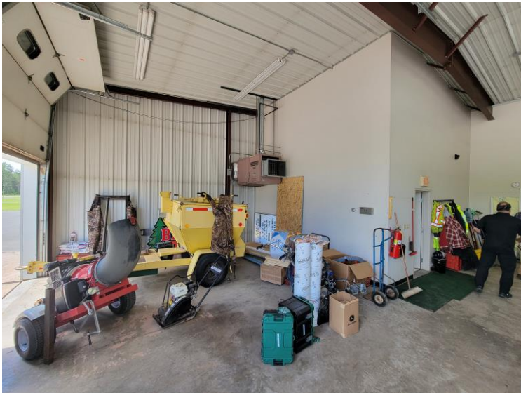
Shop, Mechanical Deficiencies
