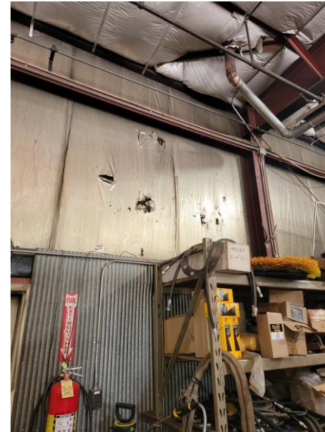
Shop, Wall Penetrations
