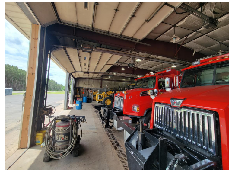
Overall Shop, Limited Height
