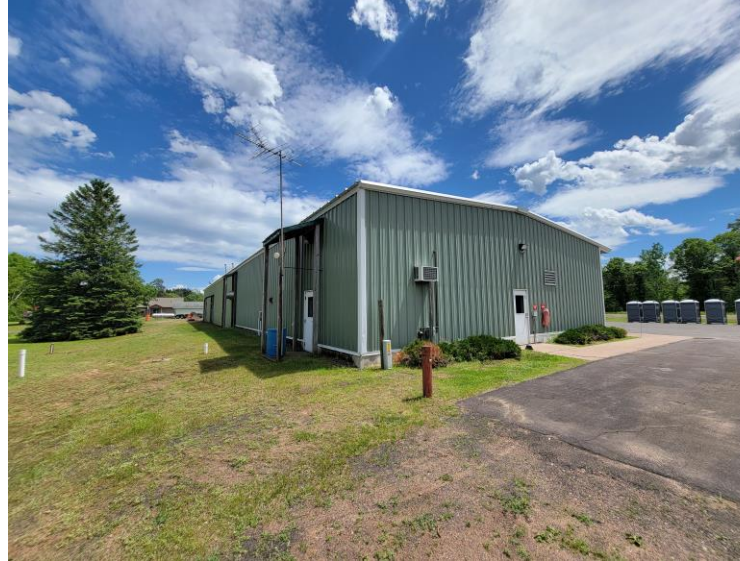
NW View, Aging Mechanical Systems
