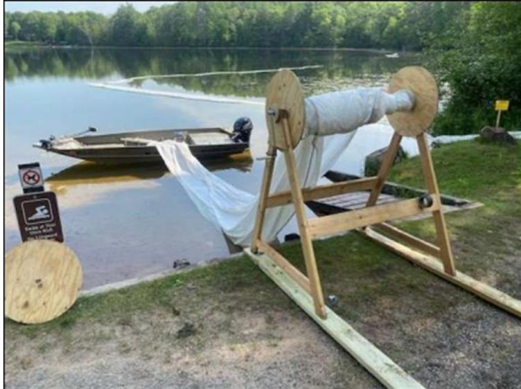
**Figure 19: Limno-curtain material on a roll before installation (photo from Marinette Co. LWCD)**
